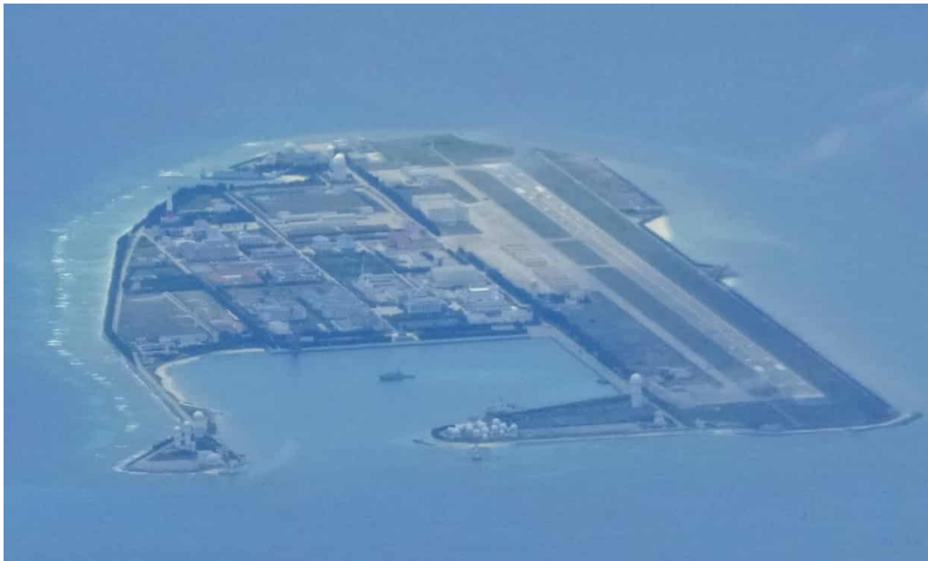
Figure 2: Chinese structures and buildings at the man-made island on Mischief Reef at the Spratly group of islands in the South China Sea (The Guardian)
